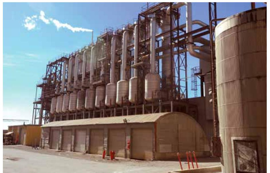
**Top: Sugar crystals growing to size inside a white sugar vacuum pan. Above: In the separator evaporation plant, additional products from molasses are thickened.** Rion Sanders photos
